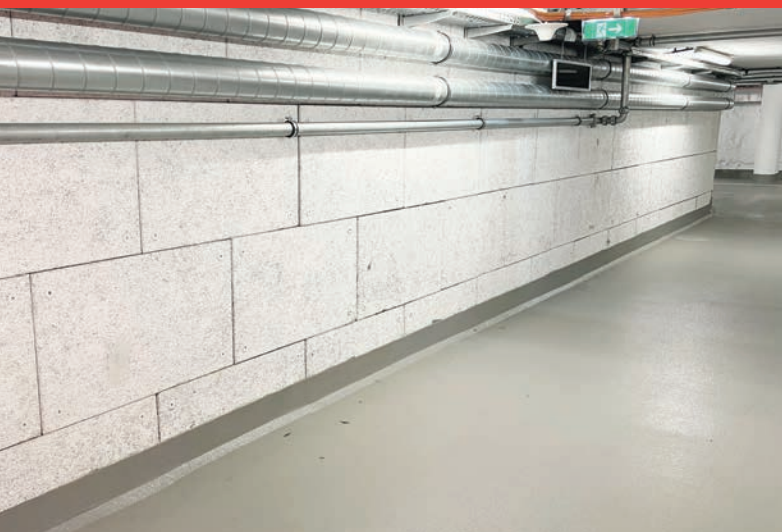
Underground garage and basement walls
