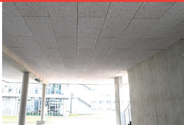
Underground parking and basement ceilings
